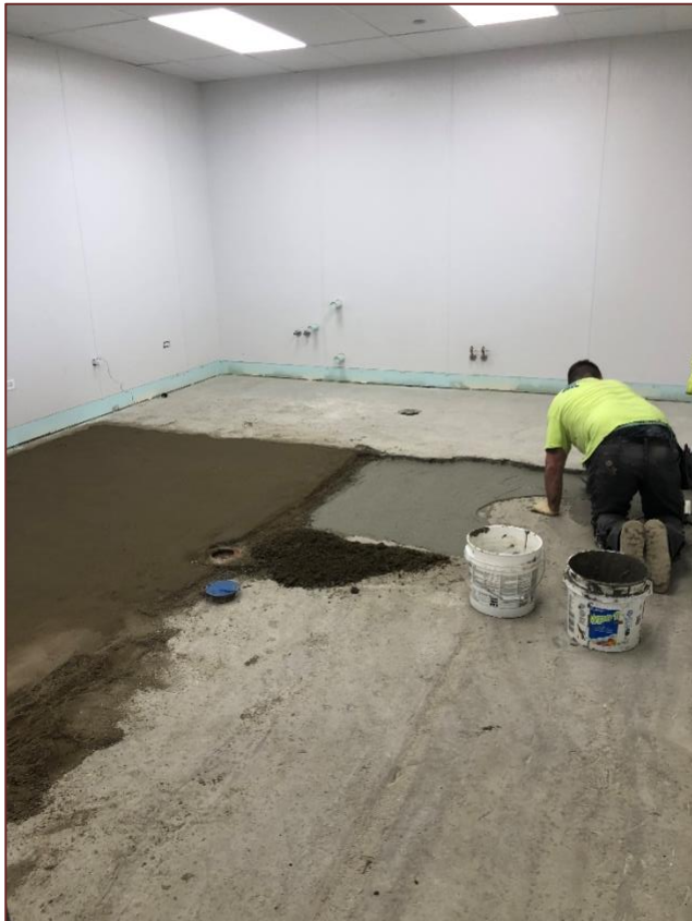
Repairing the Kitchen Floor.
