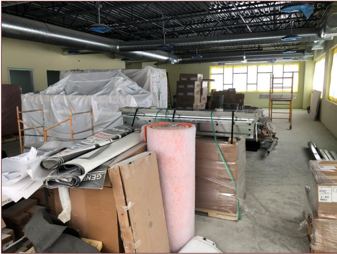
The Township Room and the delivered elevator.
