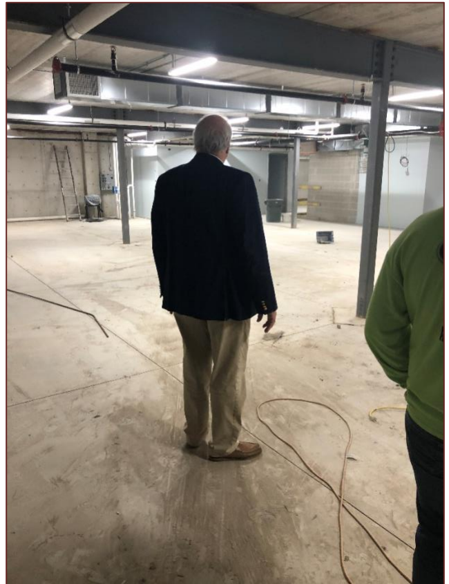
Inspecting the basement.
