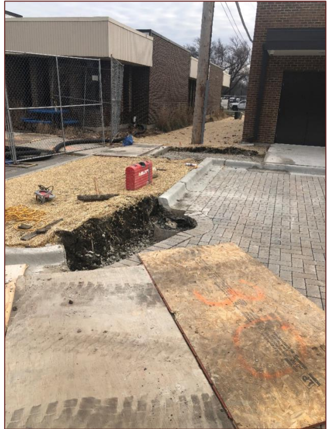
Parking Lot Work today.
