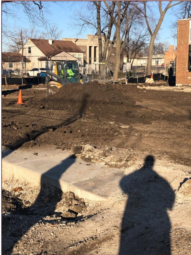
Working on the topsoil installation.
