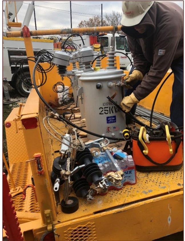
Com Ed brings power into site today.
