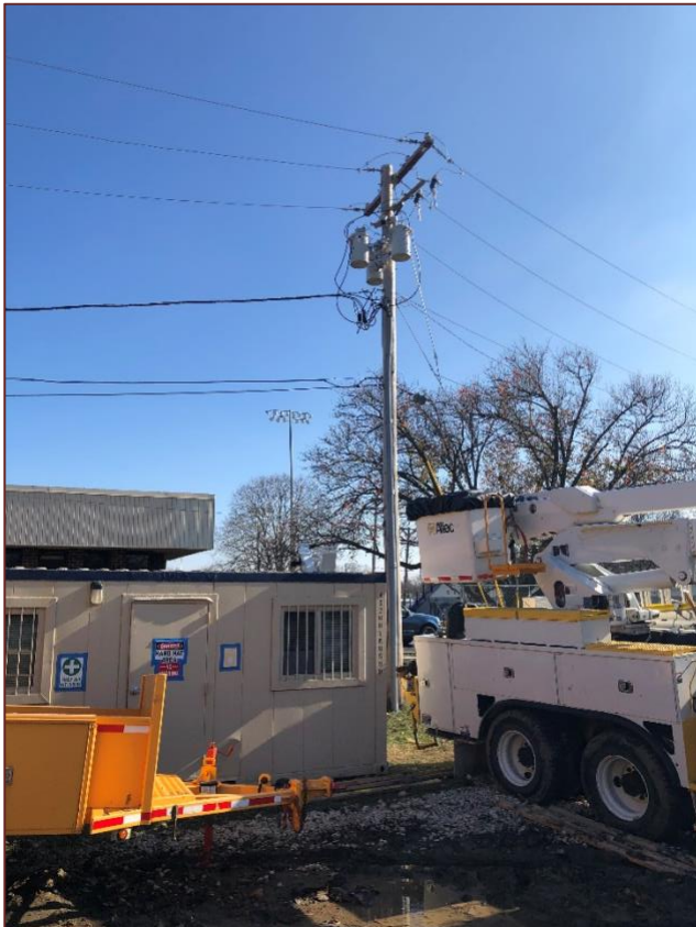
Com Ed brings power into site today.
