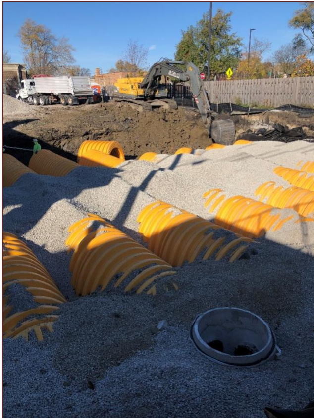
Excavation today and constructing the comp storage under the parking lot.
