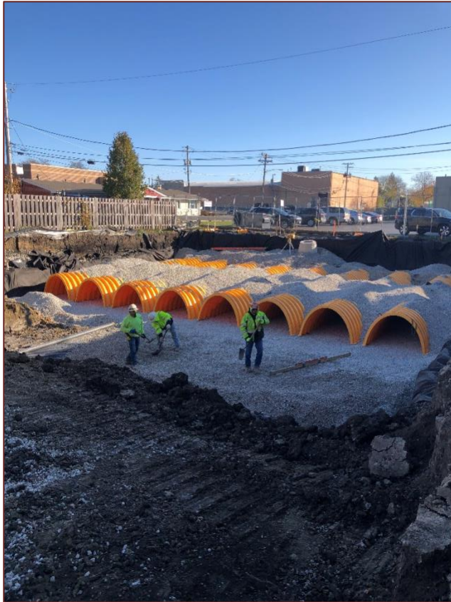
Excavation today and constructing the comp storage under the parking lot.
