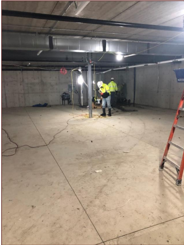
Archon works on the building water connection.
