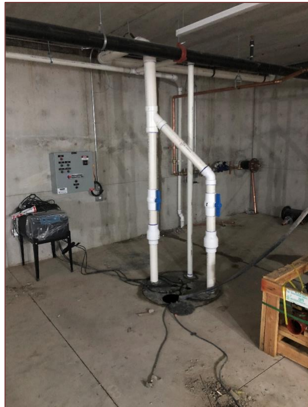
Water and sewer in the southwest corner.
