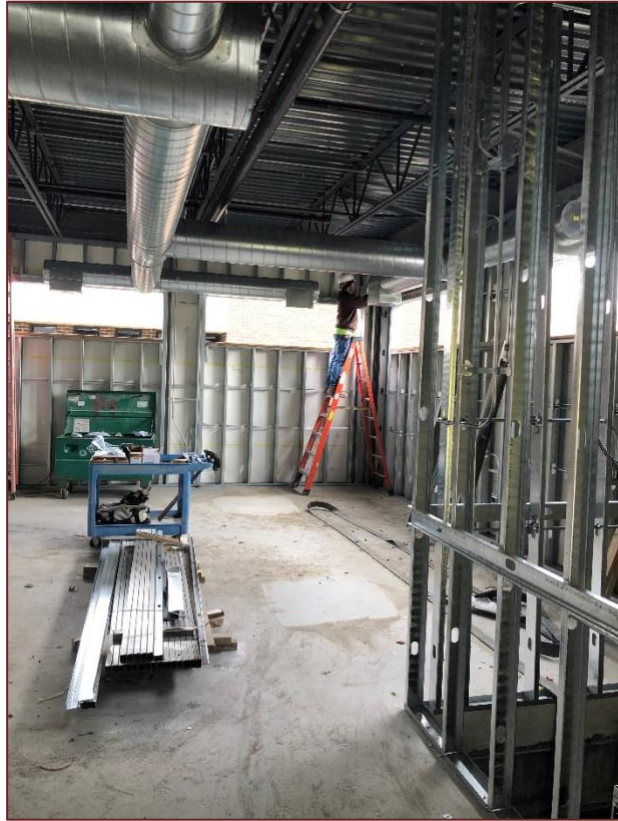
Electricians on first-floor.
