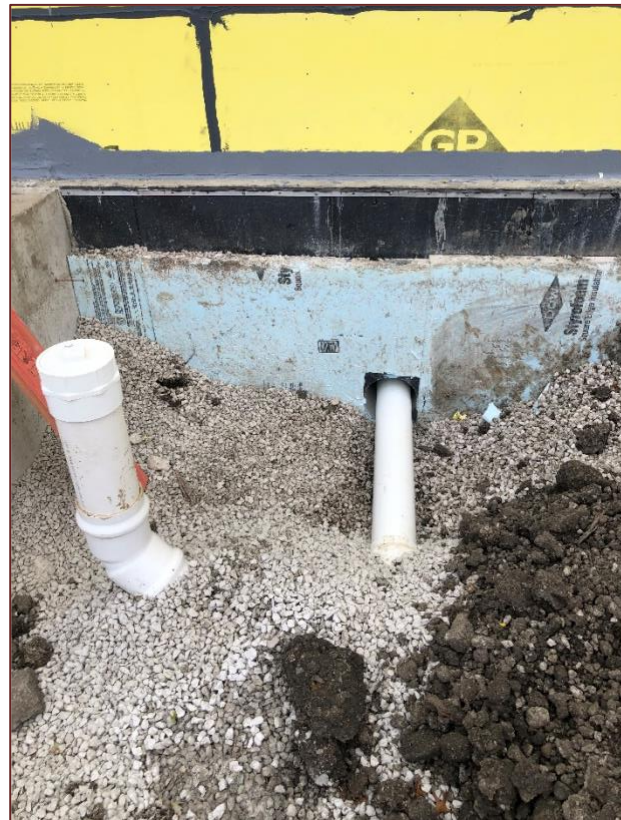
The sanitary sewer connection to the building.
