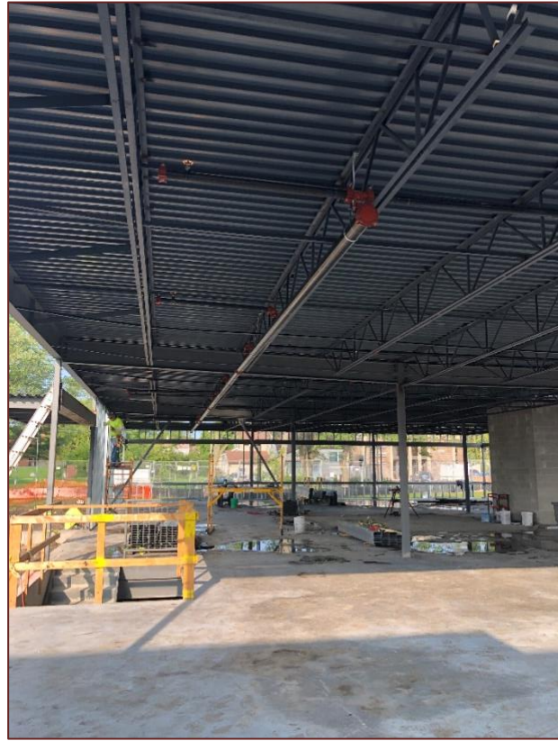
Work on first floor.
