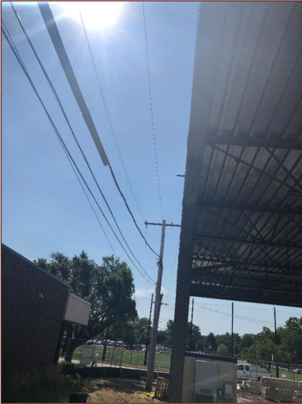
Rubbered wires.
