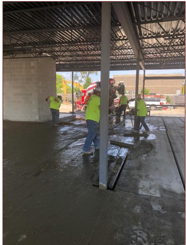
Placing the grout.
