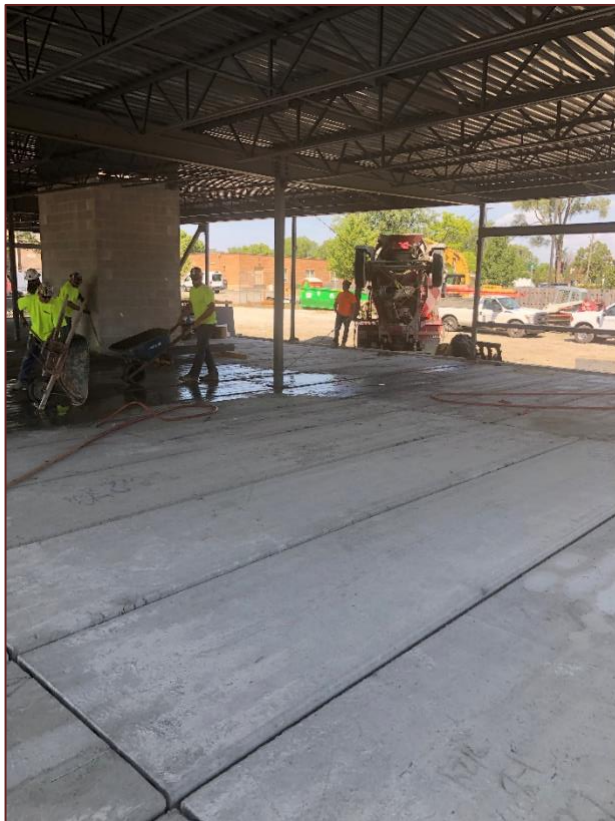
Placing the grout.
