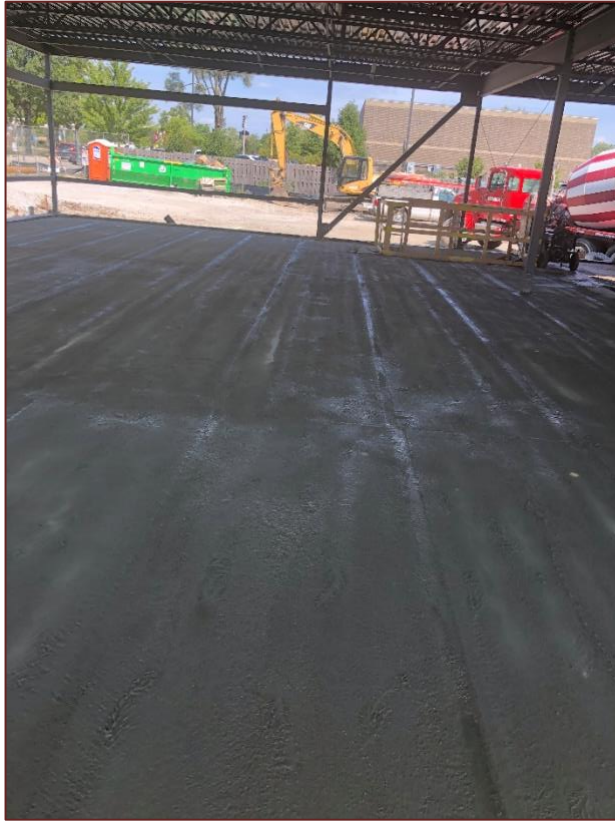
Finished grouting.
