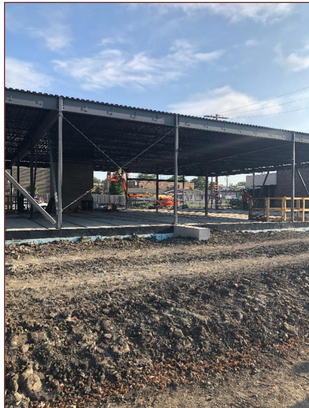
Completing the steel roofing.
