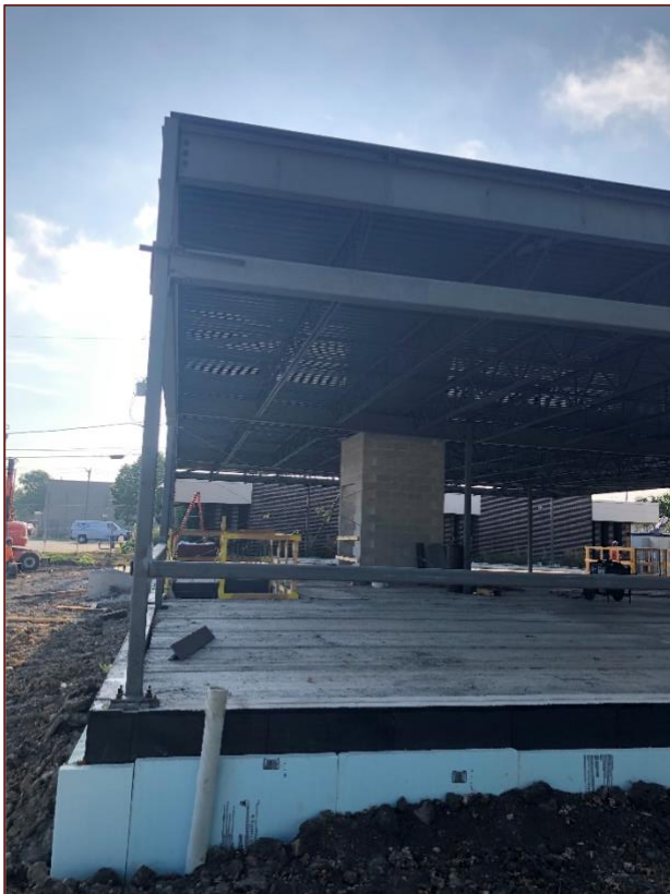
Completing the steel roofing.
