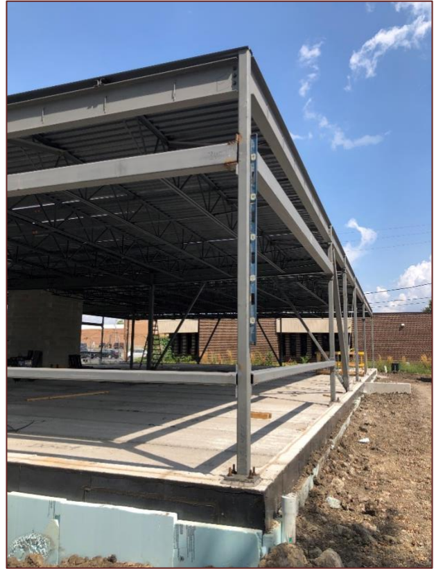
Completing the steel roofing.
