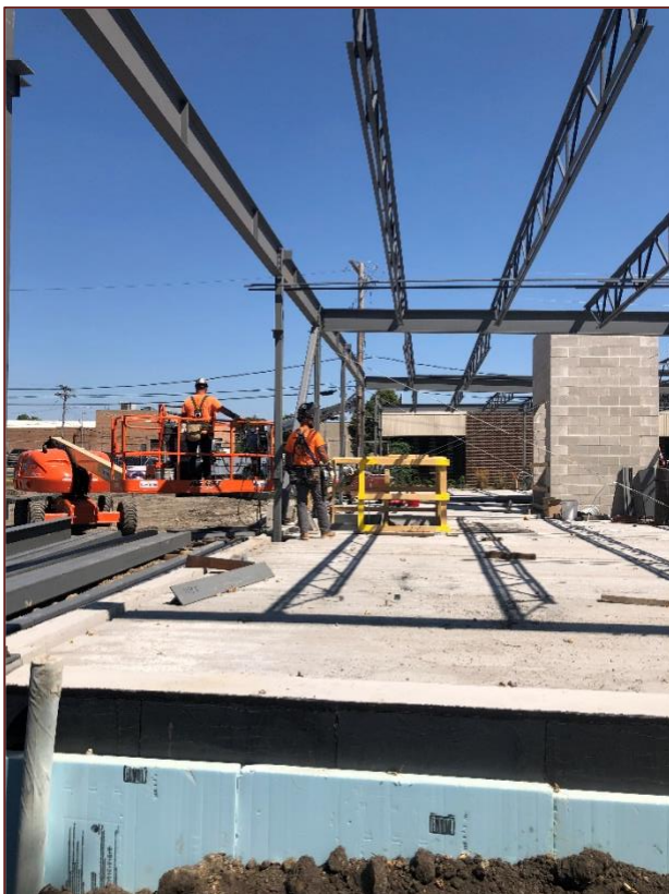
Placing steel.
