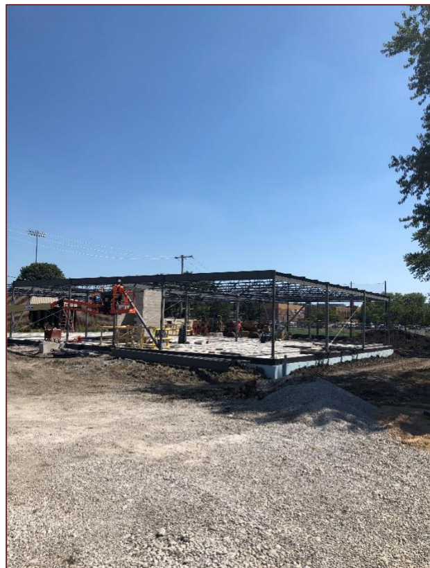
Placing steel.
