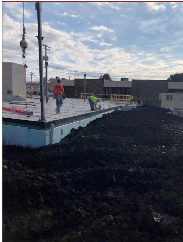
Backfilling the Walls.
