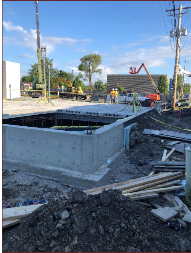
Stripping the forms from the corner walls.
