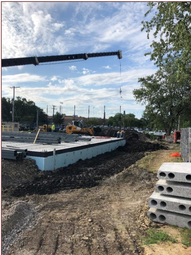
Backfilling the Walls.
