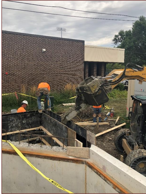
Installing the concrete.
