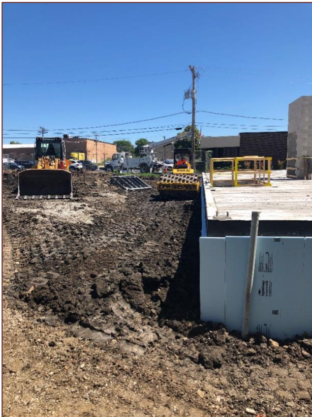
The Backfilling of the outside of the basement walls.
