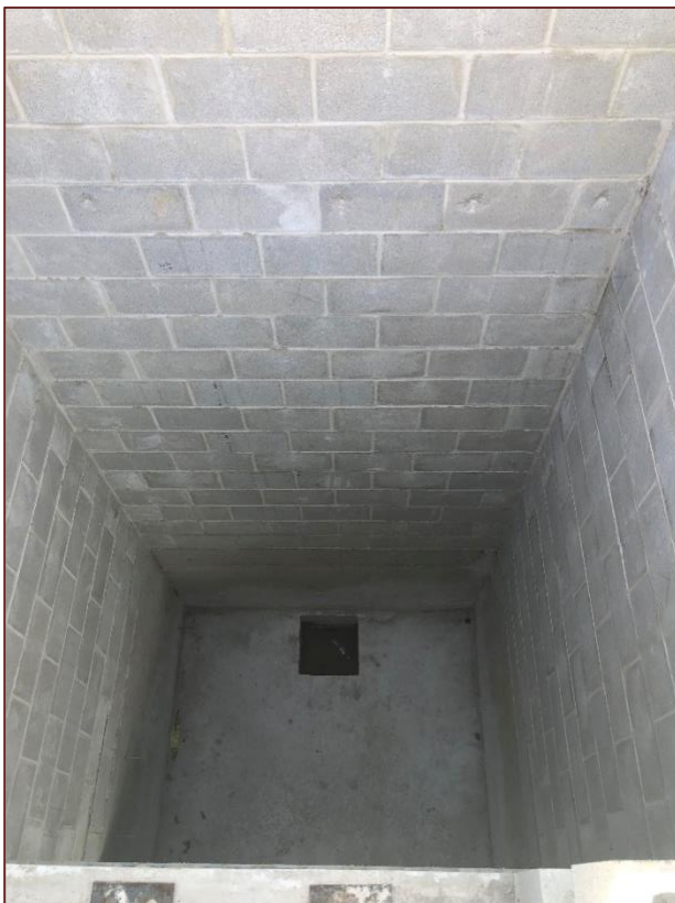
The elevator shaft.
