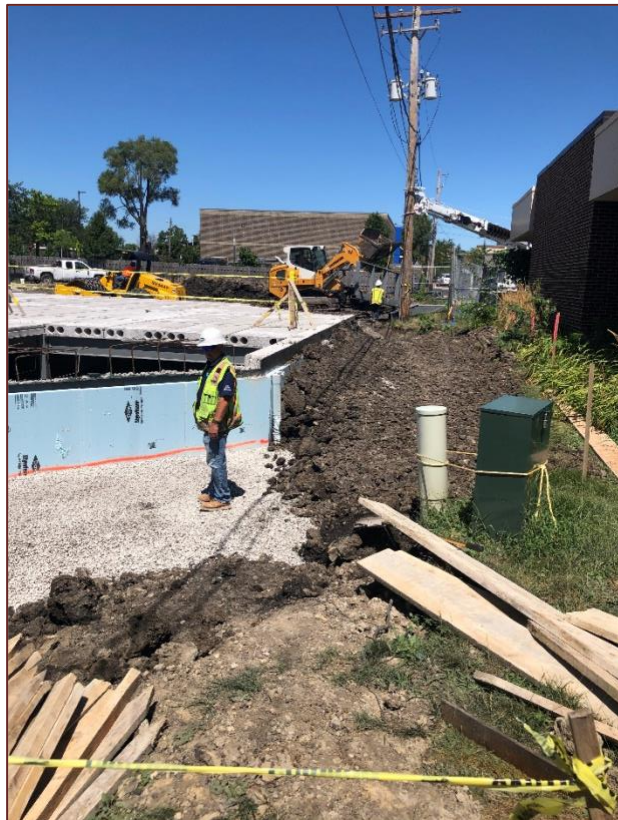
The Backfilling of the outside of the basement walls.
