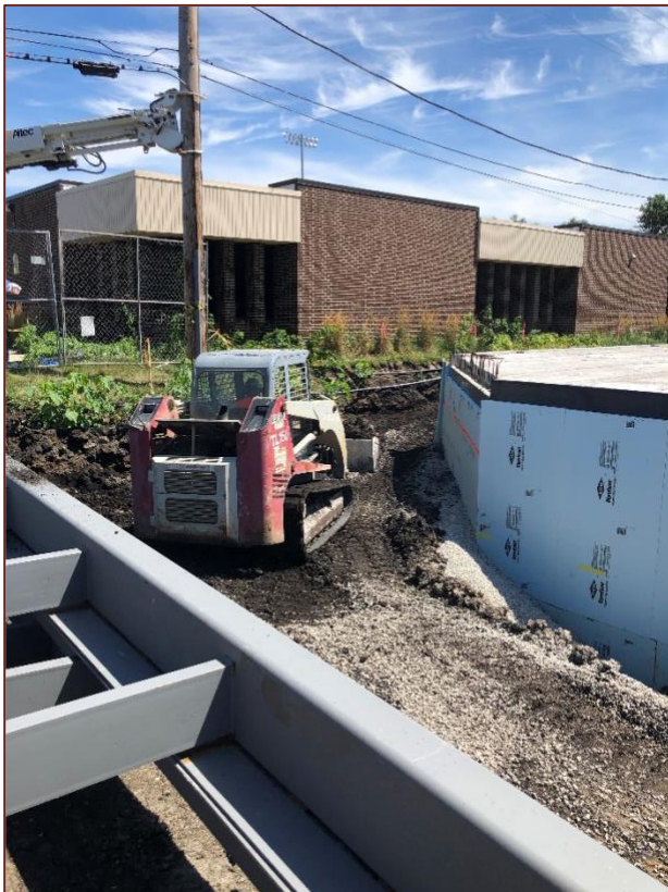
Backfilling the outside of the basement walls.
