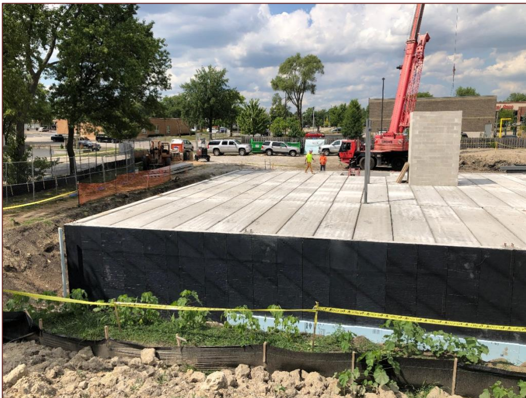
Completing the precast planks.
