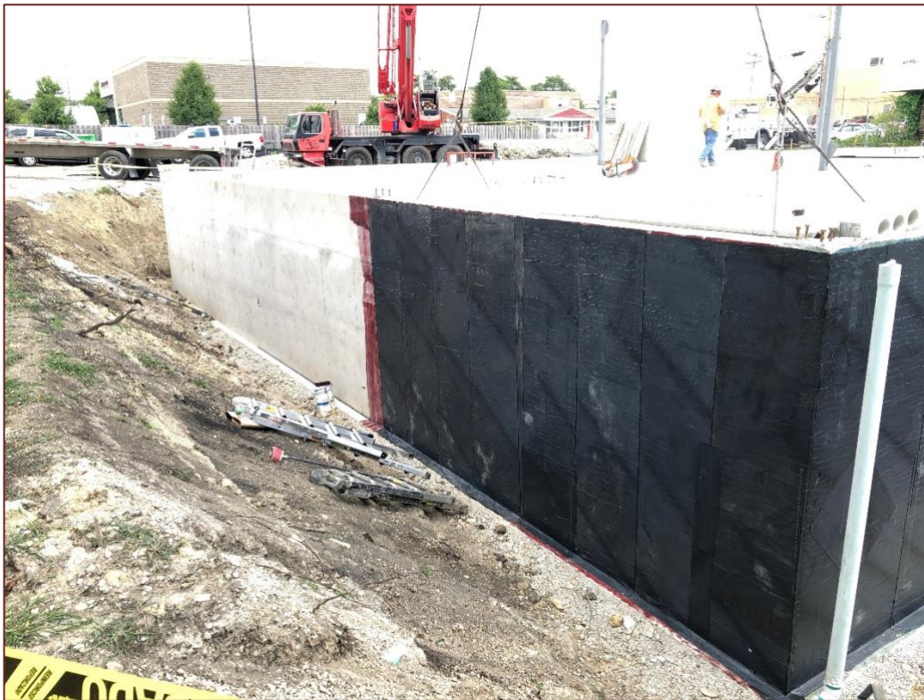
Waterproofing the walls.
