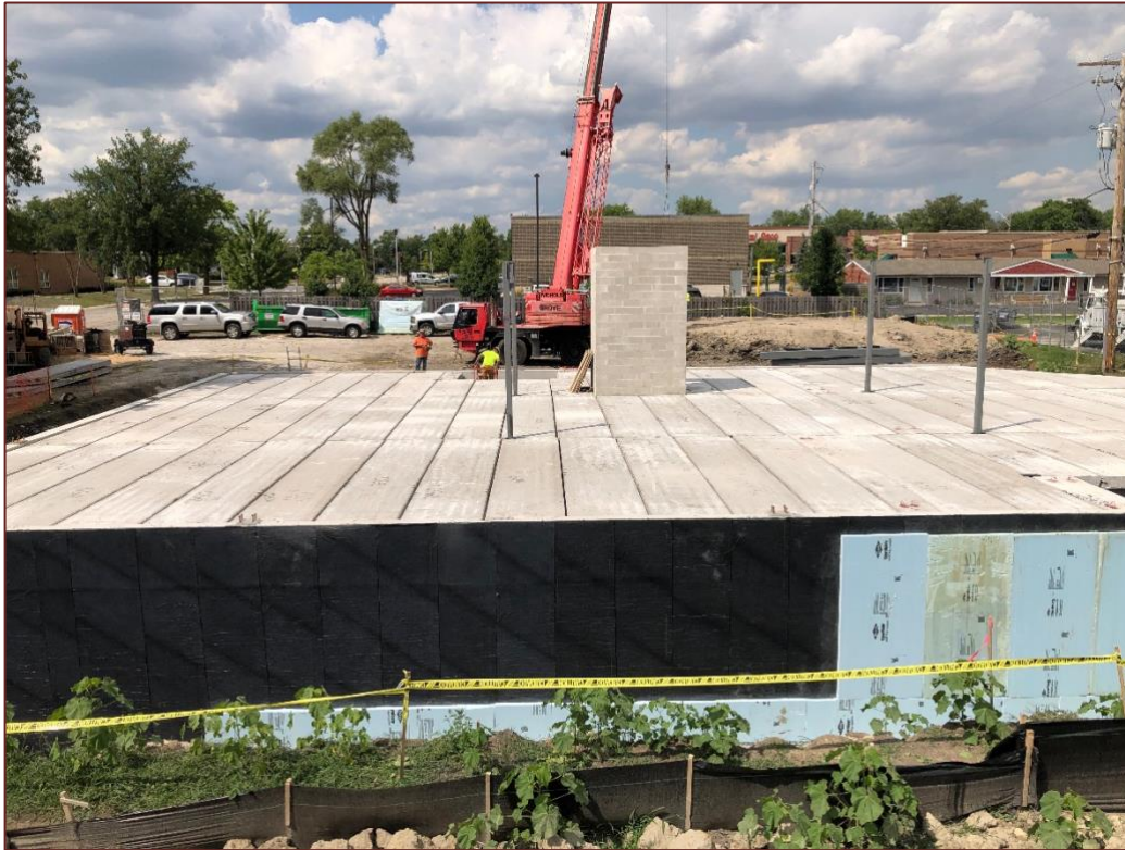
Setting the precast and waterproofing and insulation.
