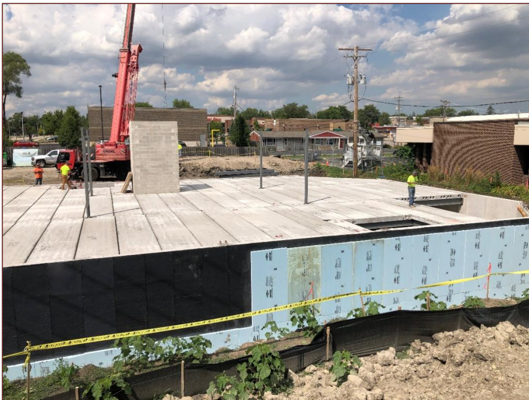
Setting the precast and waterproofing and insulation.
