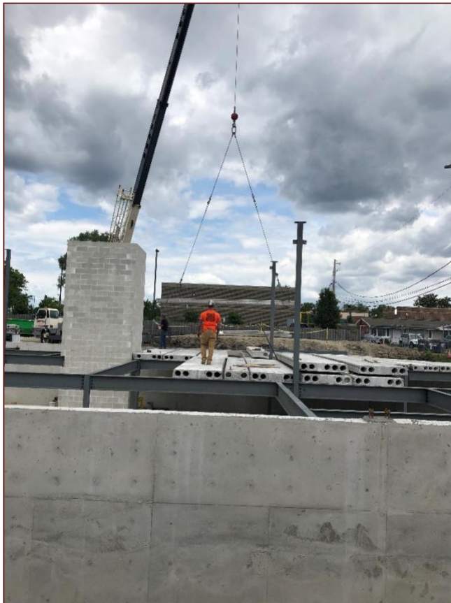
Begin setting the precast floor planks.
