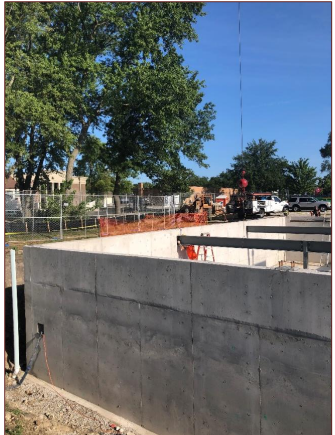
Complete setting the steel.
