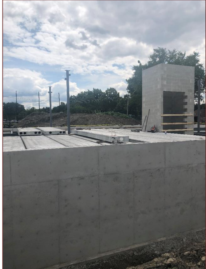
Begin setting the precast floor planks.
