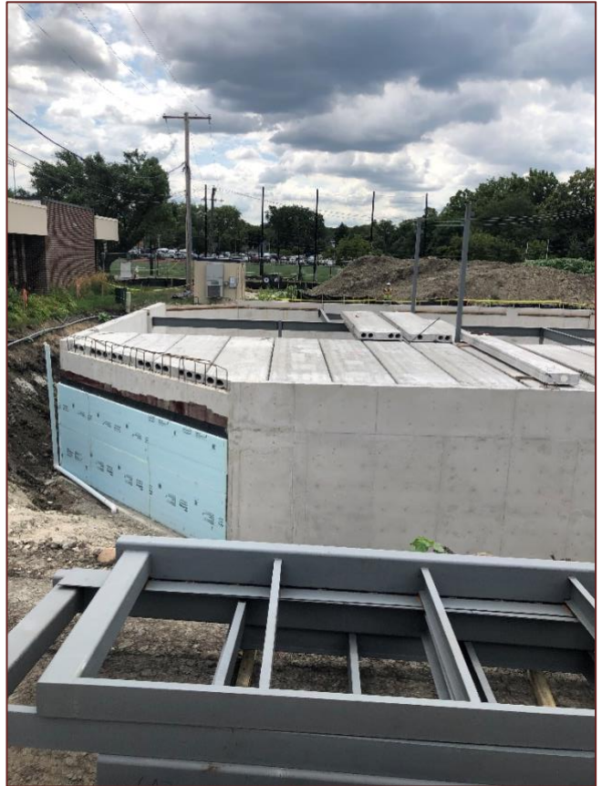
Begin setting the precast floor planks .
