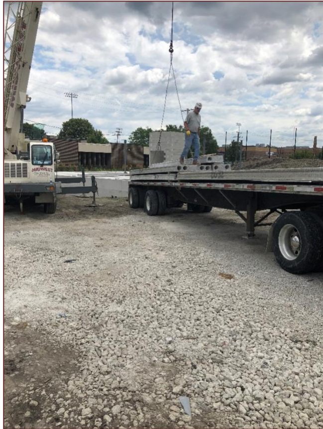
Begin setting the precast floor planks .
