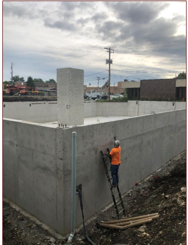
The new basement and elevator shaft.
