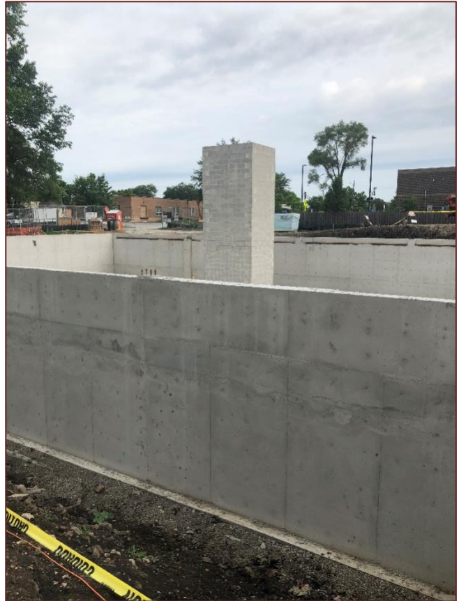
The new basement and elevator shaft.
