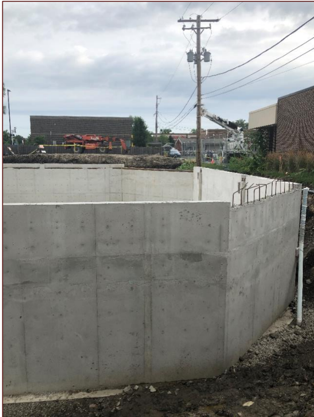
The new basement and elevator shaft.
