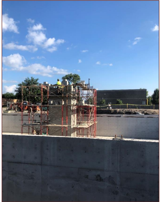
Constructing the Elevator Shaft.
