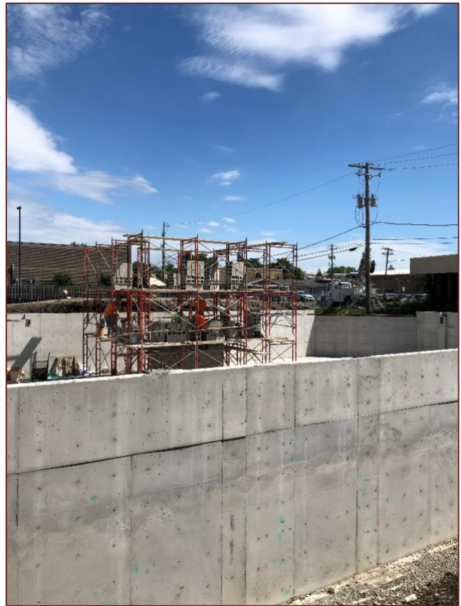
Constructing the Elevator Shaft. .
