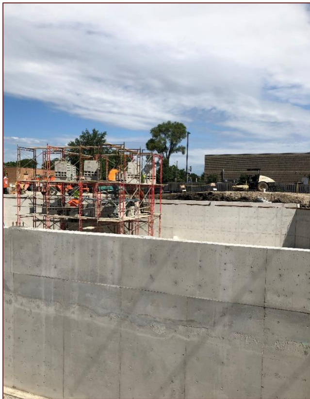
Constructing the Elevator Shaft. .
