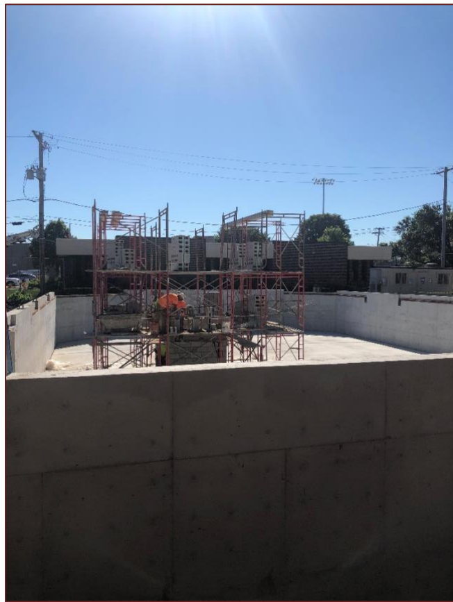
Constructing the Elevator Shaft.
