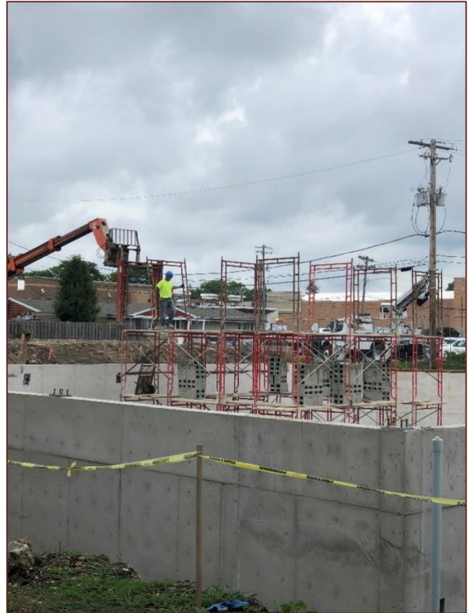
Working on the elevator shaft.
