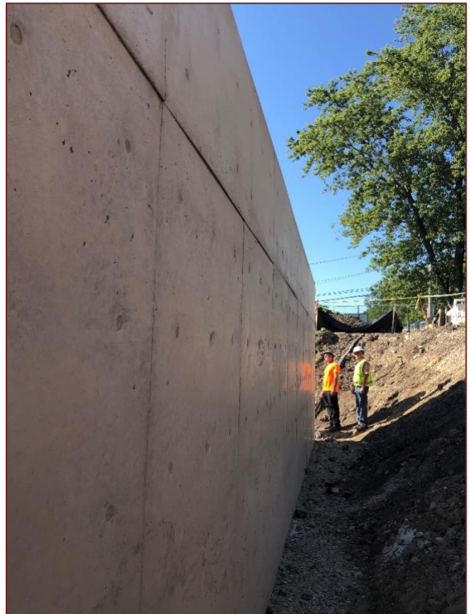
Inspecting the Basement Walls.
