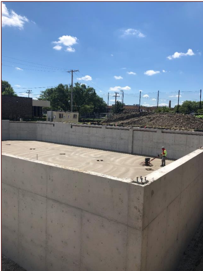
Finishing the Floor Completing the Placing.
