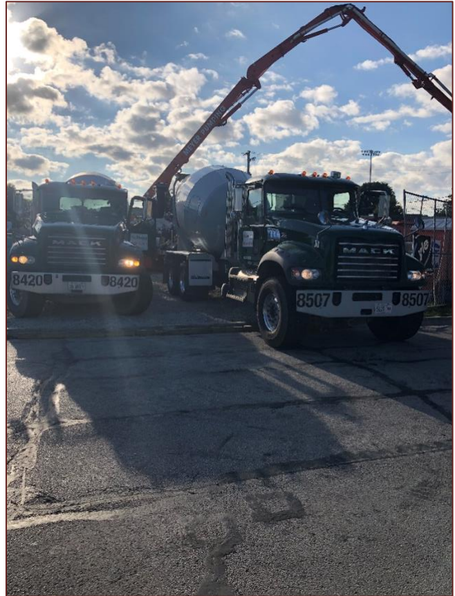
Concrete arrives at 7:20.
