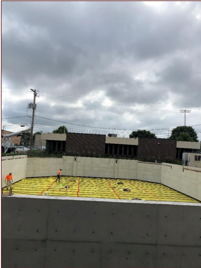
Completing the Vapor Barrier and Flooring reinforcement.
