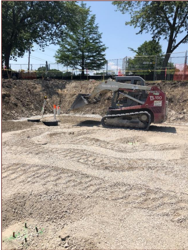
Completing the sub-base for the Basement.
