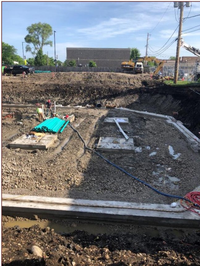
Stanton Mechanical working to complete the underdrain installation.
