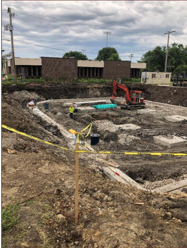
Stanton Mechanical working on the under basement piping.
